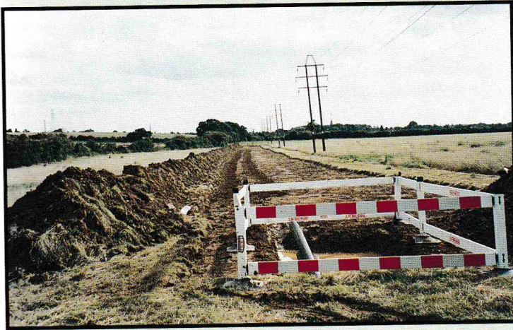
Pipeline laying to bury overhead cables.
