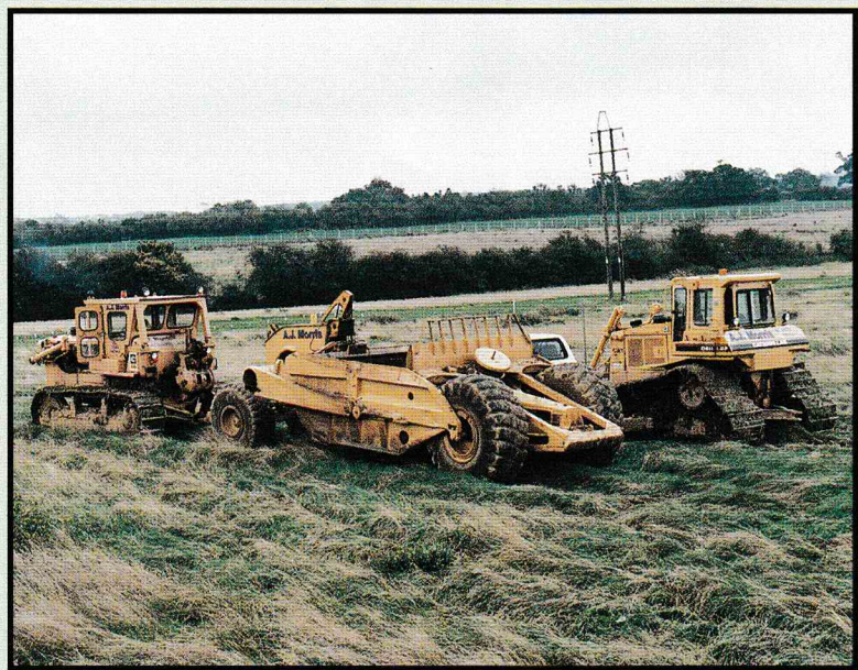
Diggers move in to start work on the lake.
